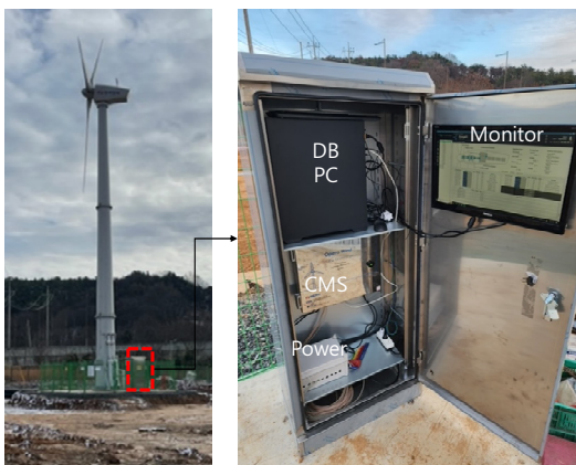
Fig. 8. Installation of data acquisition system
