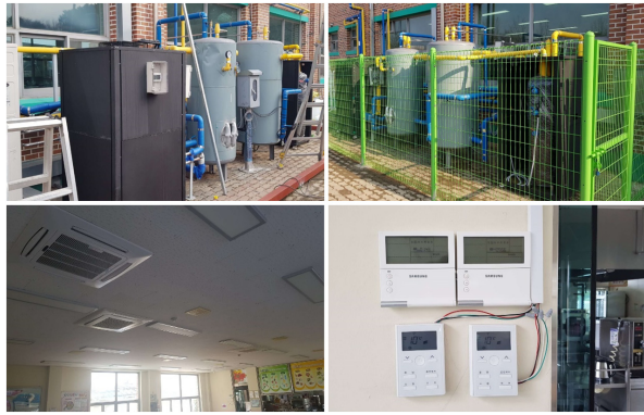
Fig. 5. Air source heat pump system
